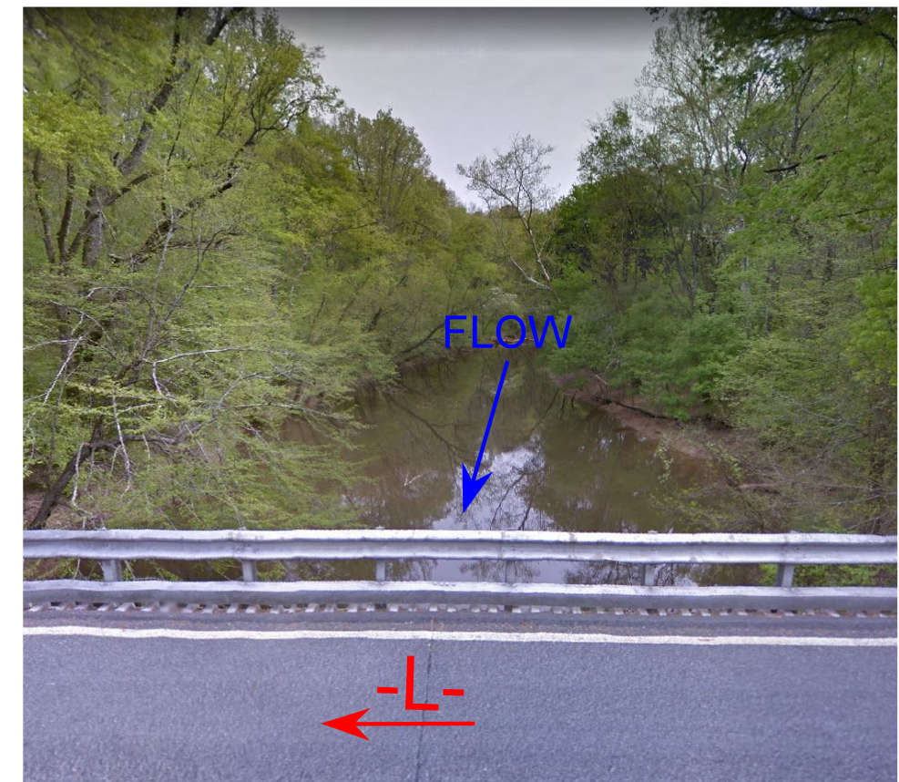
VIEW FROM EXISTING BRIDGE DECK UPSTREAM
